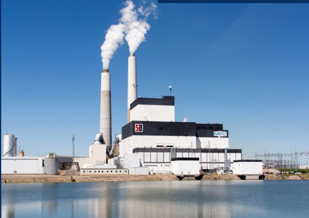
Coal-Fired Power Plant
